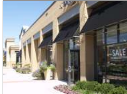
Recessed entries shall not be greater than 10 feet in depth.
