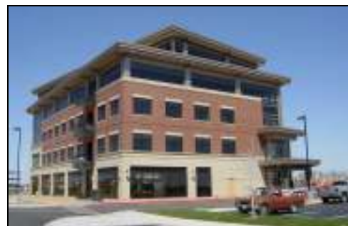
Primary front façade building materials shall be continued on side and rear façades.
