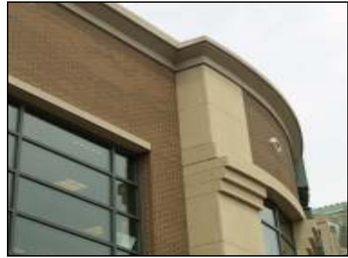
The number of materials on an exterior building face should be limited to prevent visual clutter.
