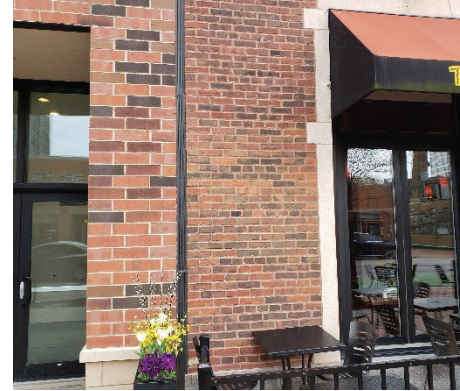
Avoid clashing building
