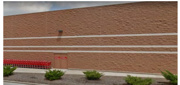
Larger bricks or concrete masonry units (CMUs) with color and texture can be appropriate for "big box" or larger buildings.
