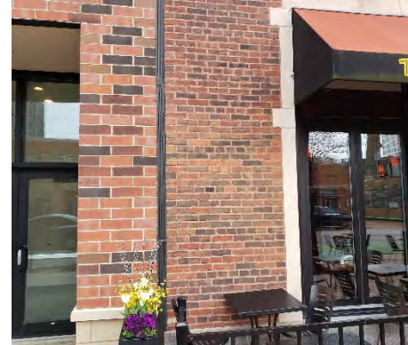
Avoid clashing building
