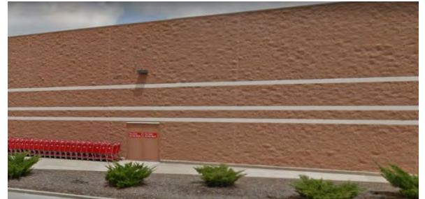
Larger bricks or concrete masonry units (CMUs) with color and texture can be appropriate for "big box" or larger buildings.
