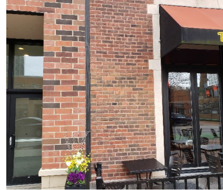
Avoid clashing building
