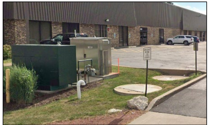
Figure 1 - Klefstad Lift Station
