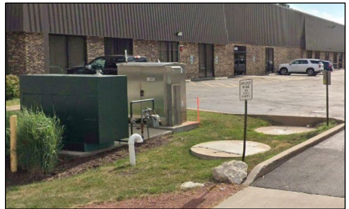
Figure 1 - Klefstad Lift Station
