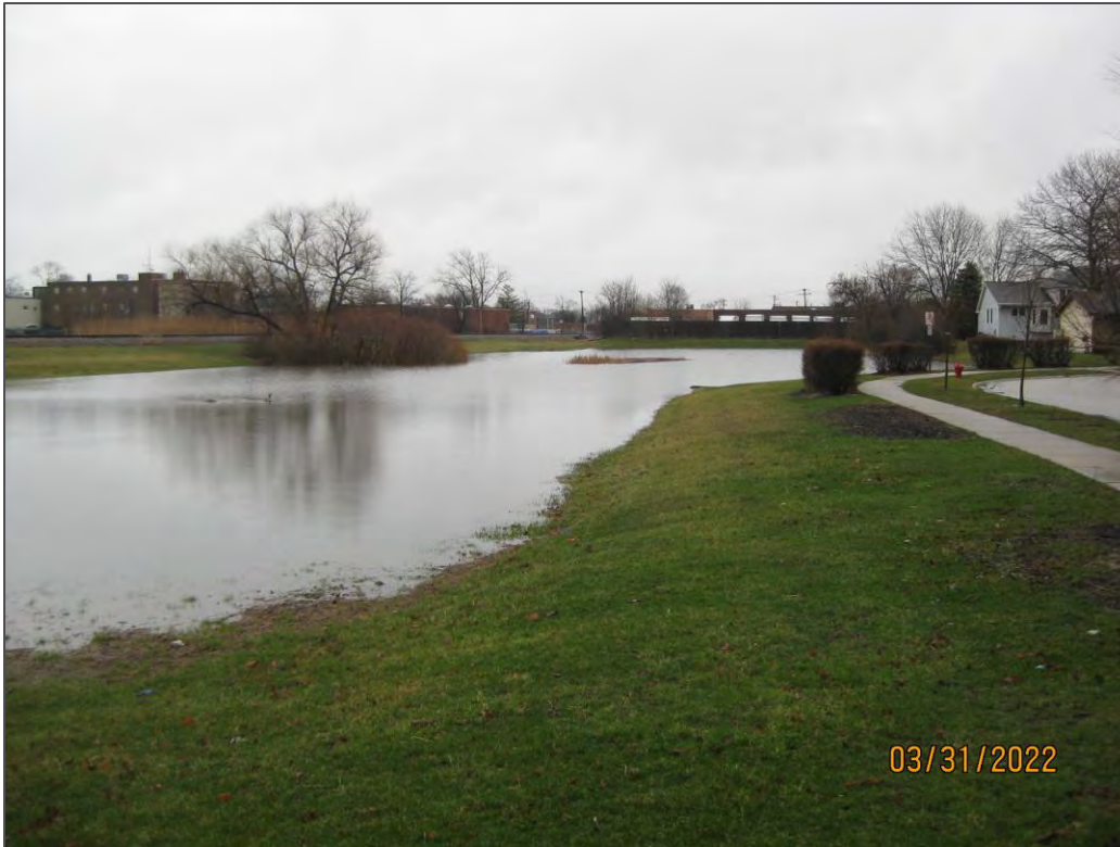
Figure 5: The existing basin after a rain event on March 31 st , 2022. The City received 1.25 inches of rain on this day. Stagnant water remains for long period of time since the basin does not drain properly.
