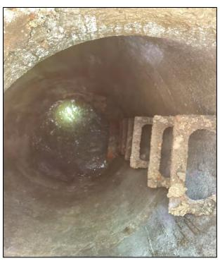
Figure 4 – Discharge Manhole Corrosion
