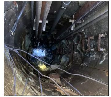
Figure 2 – Cementitious Liner Deterioration
