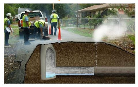
Non-toxic smoke testing is performed by blowing harmless smoke into a sewer segment through consecutive manholes at both ends of a pipe. Defects are identified where smoke exits the ground or structure. Smoke testing identifies sewer system openings that allow rainwater to enter the sanitary sewers. Commonly identified concerns include leaky manholes, cracked main lines and laterals, downspouts, storm sewers,
