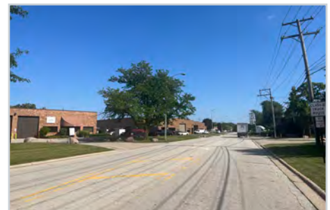
Current Conditions of Central Avenue
