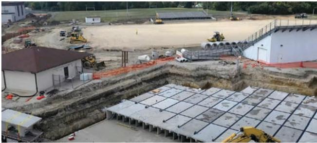
The tank is complete and almost all of the new pipes are installed. We are now largely focusing on the installation of new artificial field turf. This incredible opportunity is a byproduct of needing to replace stormwater pipes inside the stadium. Once completed, we can bring soccer home to Fenton for the first time in decades. We can also have multiple teams, clubs, and classes use the field every day without pausing to let grass regrow.
