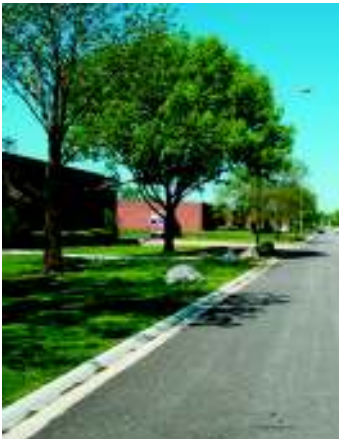
Pedestrian connections, sidewalks, and bicycle facilities are missing in many locations
