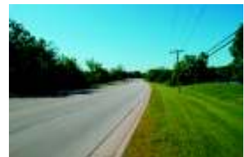
The Study Area is in good physical condition
