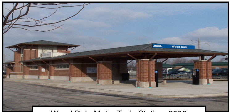
Wood Dale Metra Train Station, 2009
