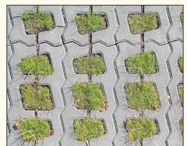
Rain barrels store stormwater which can be used to water gardens and lawns, while permeable pavers decrease runoff by allowing water to percolate through the pavement's surface.
