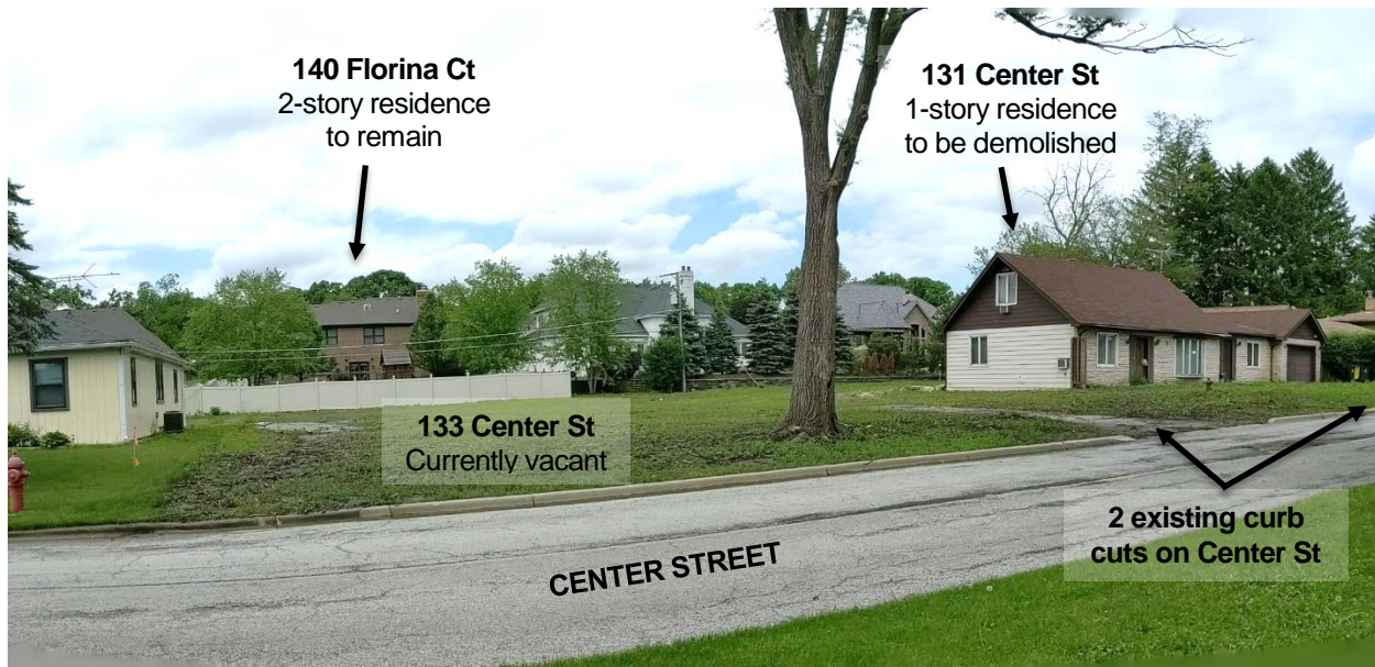
View 131-133 Center Street looking north
