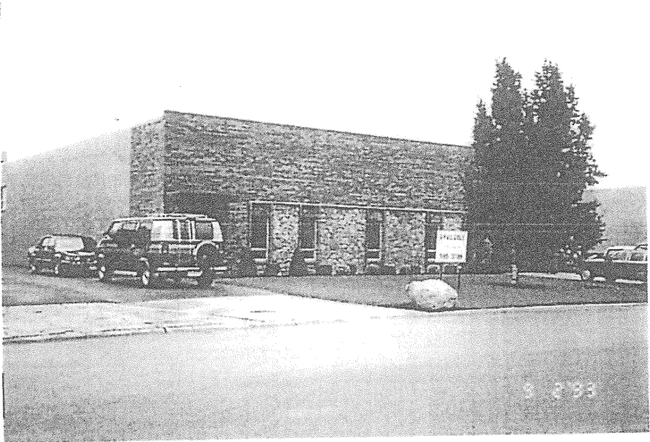
Front of subject structure from across Lively Boulevard.
