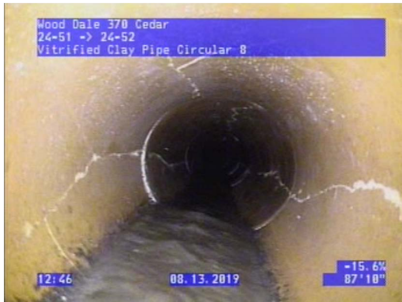
Crack Hinge 87.8'
