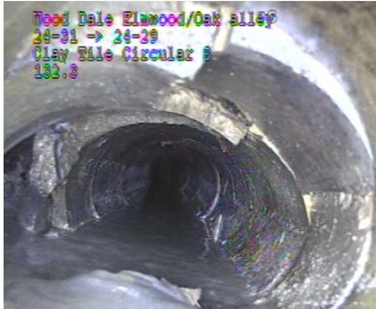
Severe Root Infiltration MSA 172'
