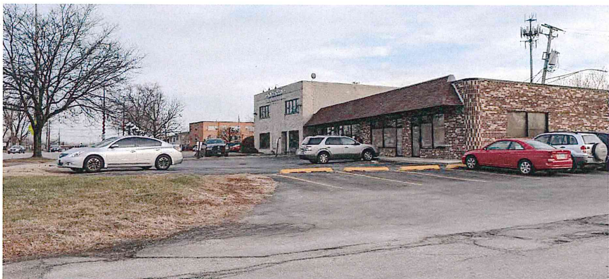
View of subject property looking south-east from Edgewood Ave
